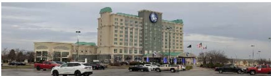
Isle Casino & Hotel - Waterloo
