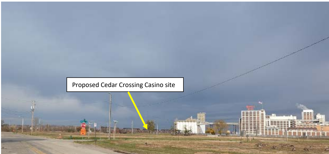
View to the north looking across proposed casino site
